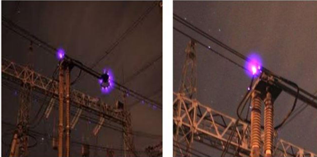
. Figure(3.12) The corona effect in transmission overhead line.
