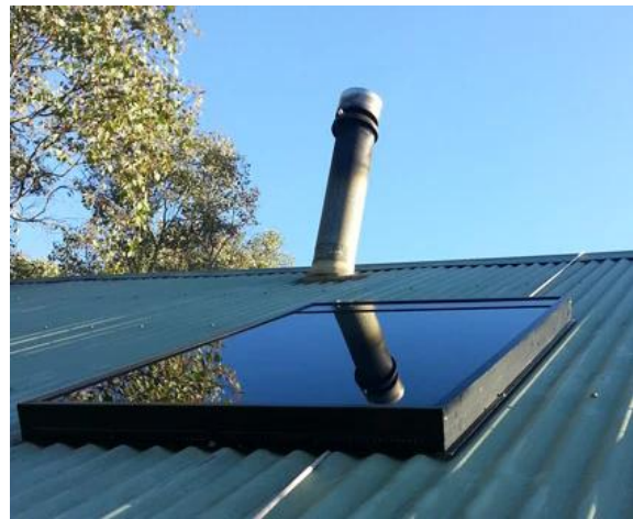
Figure (1-1) solar air heater.
