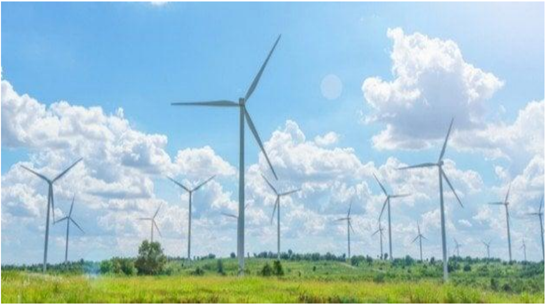
Figure-2. Wind farm consisting many wind turbines.
