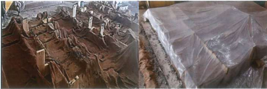
Figure 3.28 Beams Curing.
