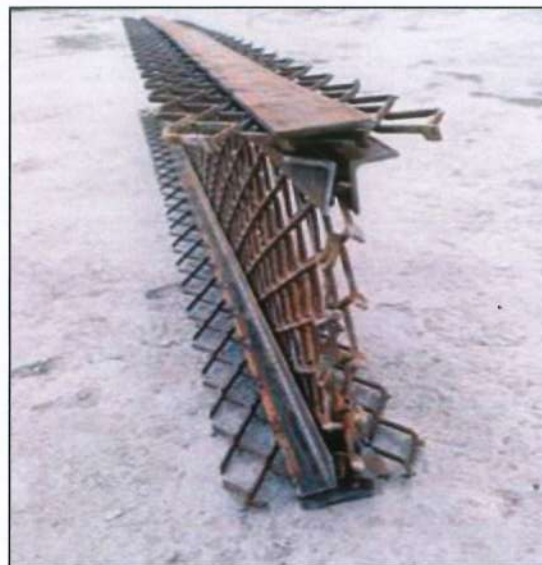
Figure 3.21 I- Shape Shear Connector.
