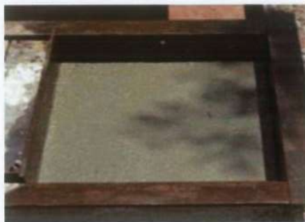
(a) Casting of Bottom Wythe
