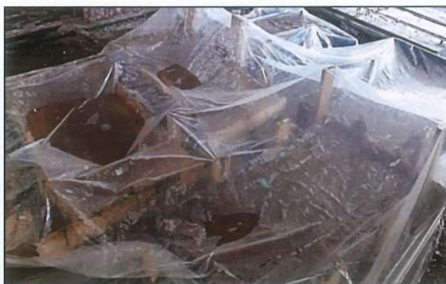
Figure 3.36 Curing for Panels.
