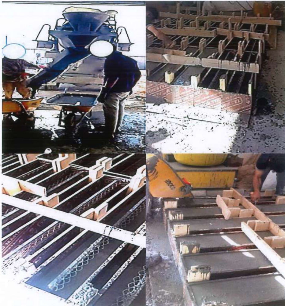
Figure 3.27 Casting of the Beam Specimens.
