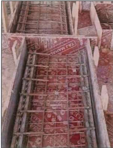
(a) Installing reinforcement and connectors.
