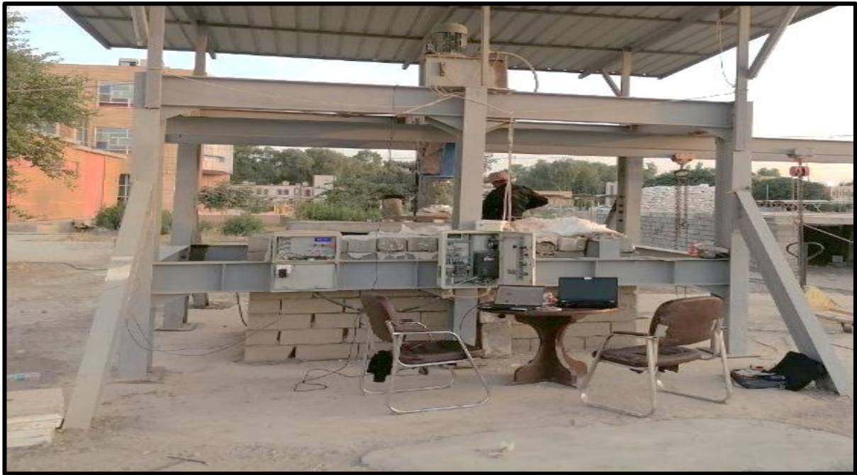
Figure 3.17: The outer iron structure of the furnace
