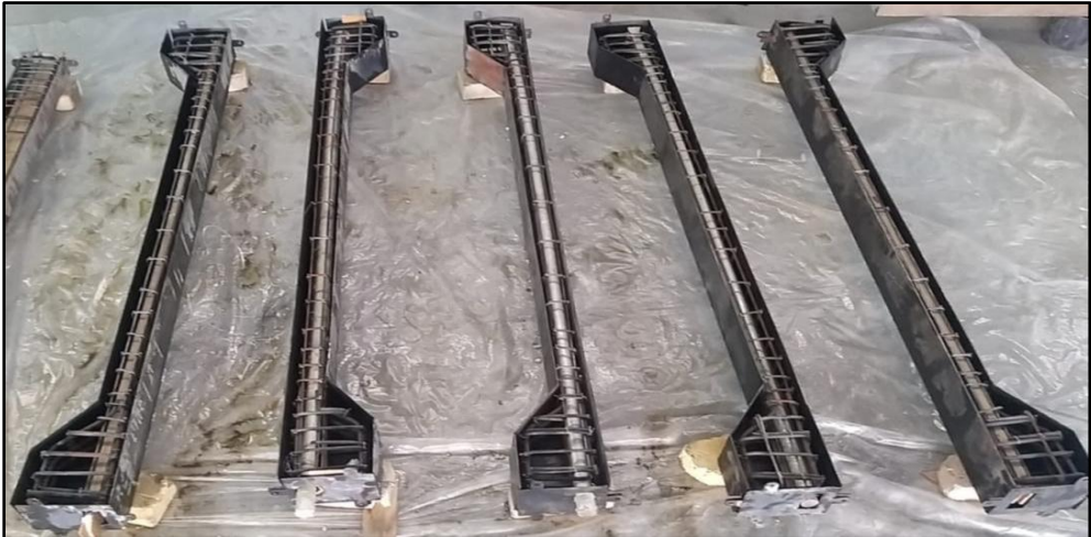
Fig. 3.17 Steel Reinforcement cage and mold with corbel.
