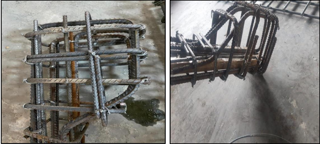
Fig. 3.18 The reinforcement of corbels.
