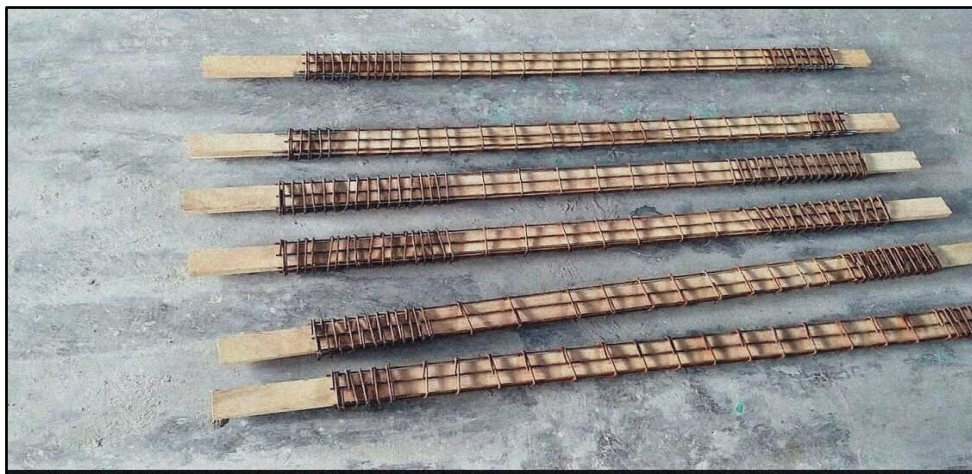
Fig. 3.15a Cage of steel reinforcement for columns (C1-C7).
