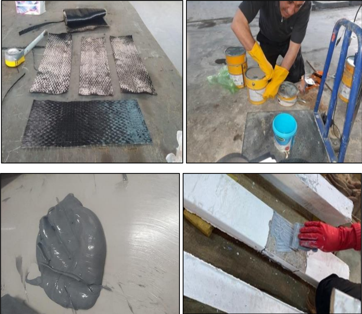
Fig. 3.33 Steps of installation CFRP sheet
