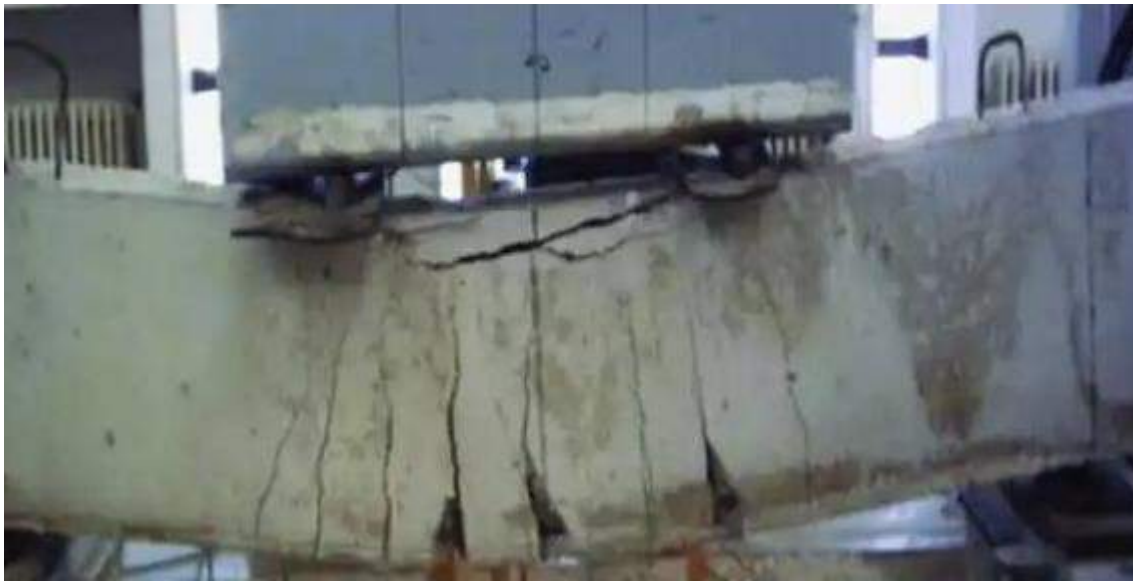
Figure 1.3 Flexural Failure in Beam
