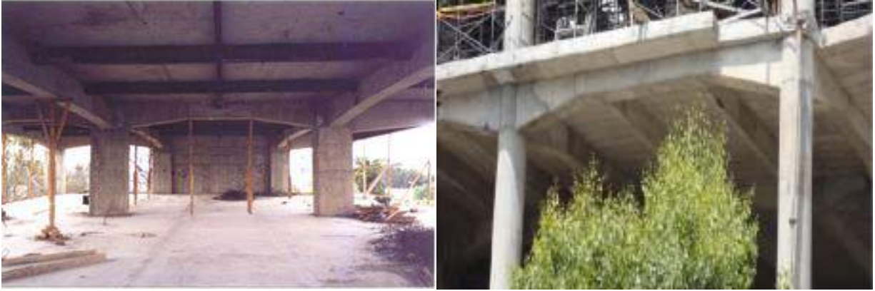
Figure 1.2 RC buildings with hunched beams recently constructed in Mexico City[4] .
