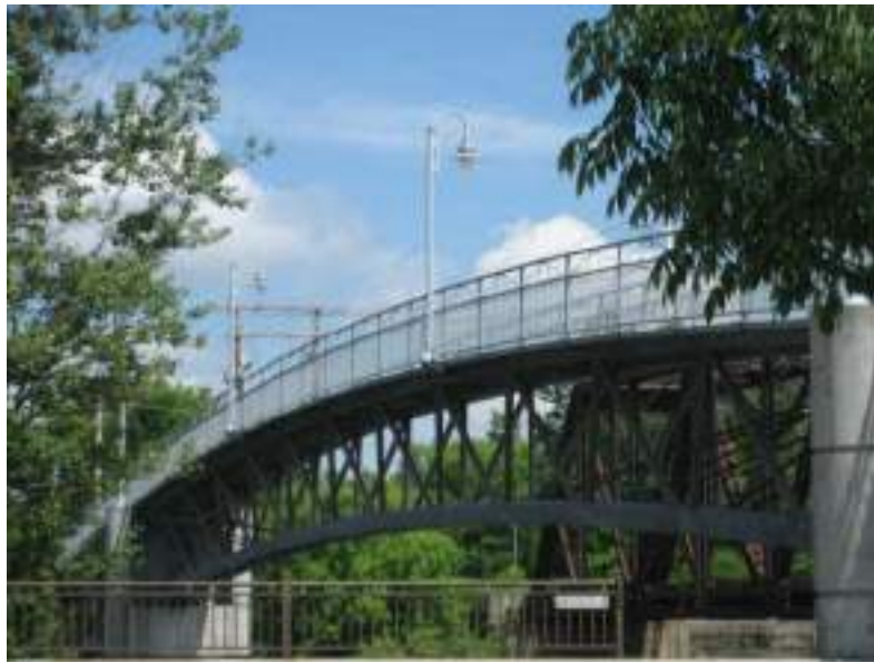
Figure 1.4 Sherbrook Pedestrian Bridge, in Canada.
