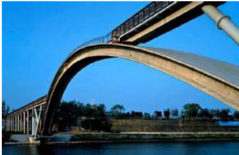
Figure 1.5 Seoul Footbridge in South Korea.
