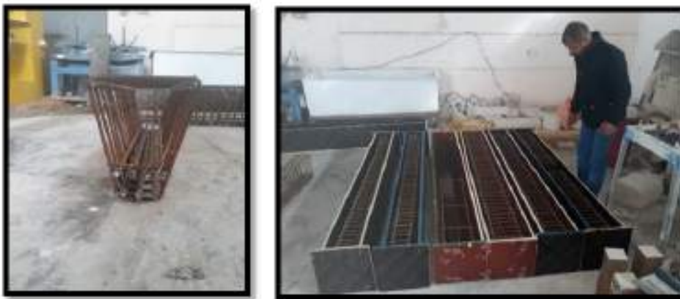
Plate (3.6) Fabrication and installation of reinforcing bars
