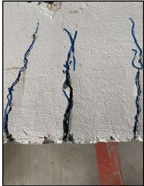
Crack Width
