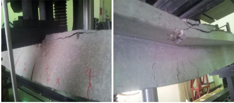
Figure 2-1 Crack pattern and shape of triangular and T-beams after collapse [33]
