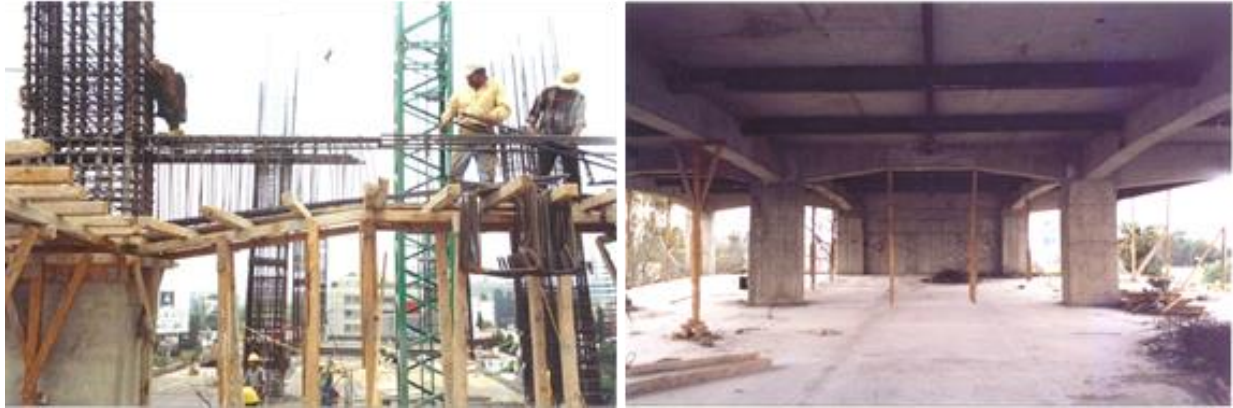
Figure 1-6: RC buildings with haunched beams recently constructed in Mexico City [18]
