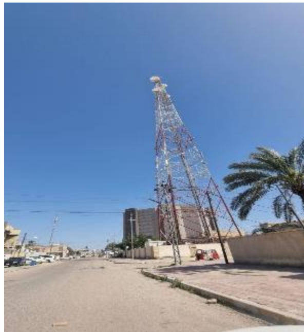
Figure 3-10. UMTS for Site 1.
