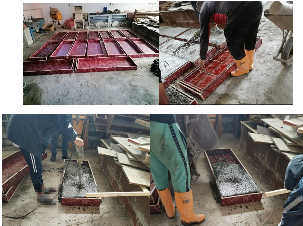
Figure 3.18 The Details of Slabs Casting.
