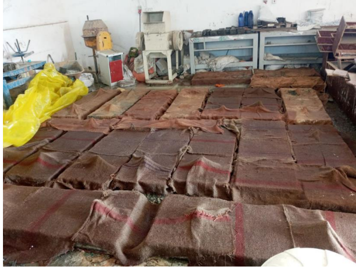
Figure 3.19 The Curing of Slabs.
