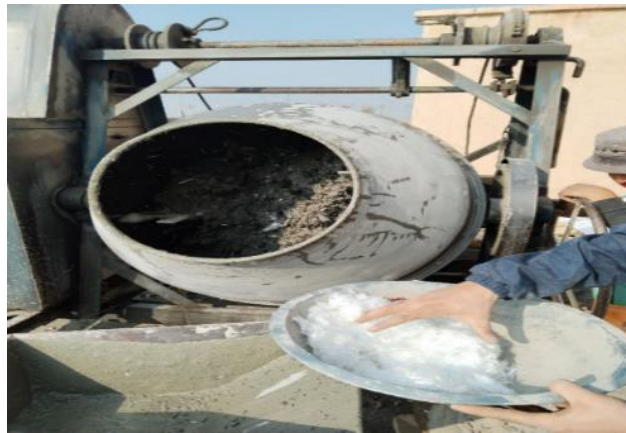
Figure 3.7 Manually Adding Fibers to The Mixer.
