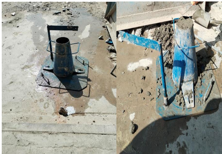
Figure 3.9 Slump Test for Concrete.
