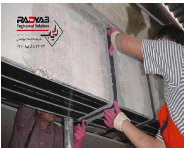
a) EBR sheet in the external surface
