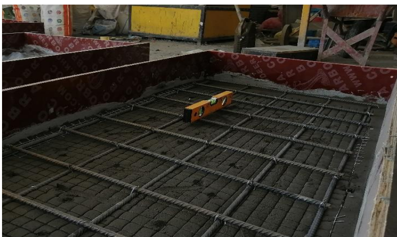
Figure 3.14 Rebar on the top surface of cover
