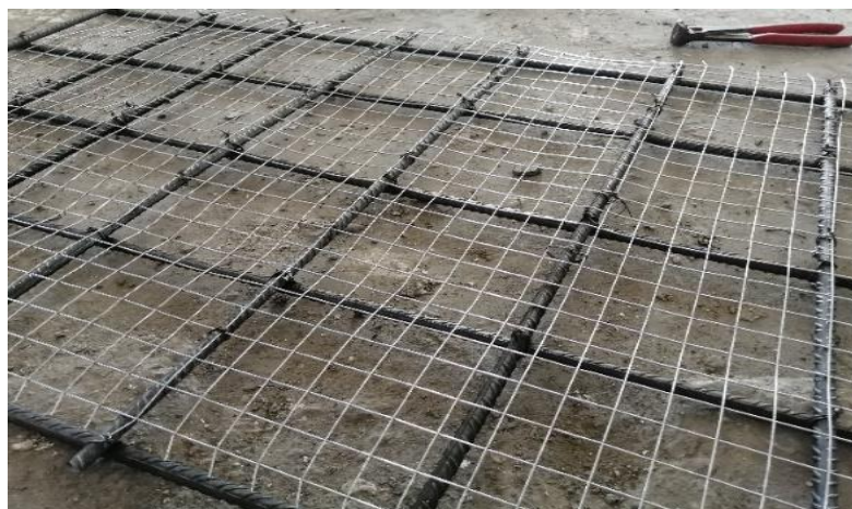
Figure 3.13 wire mesh connect with rebar
