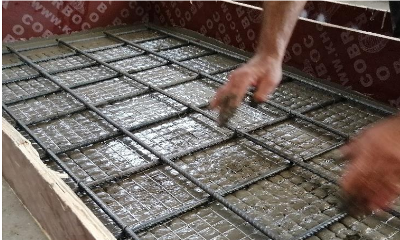
Figure 3.12 Embed the wire mesh
