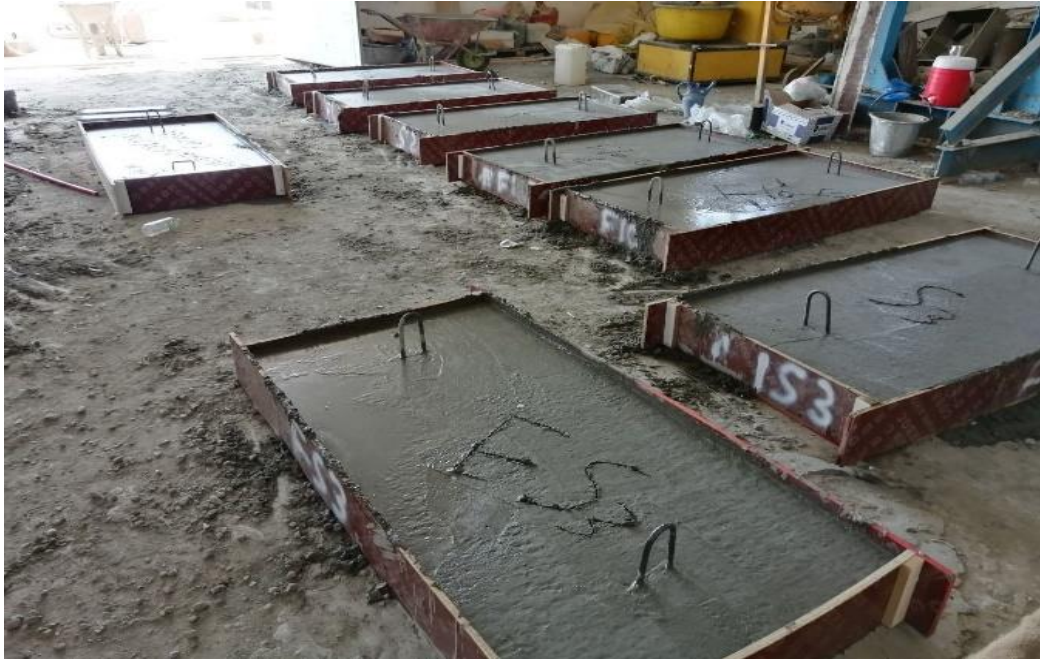
Figure 3.18 Casting of the specimens
