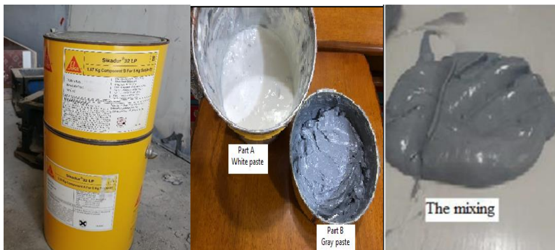
Figure 3.1 Mixing epoxy components (Sikadur-32LP)
