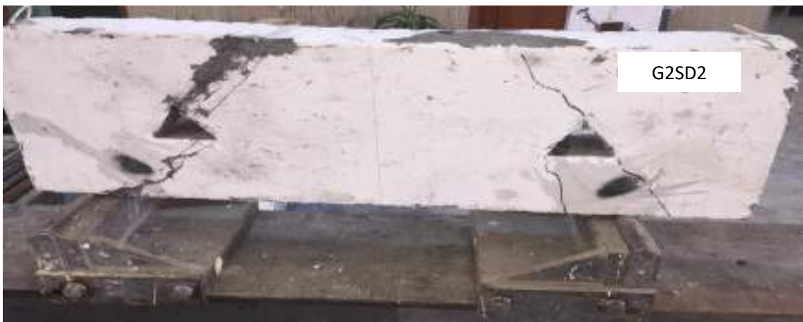
Plate (4.34) Experimental Deep beam G2SD2 (9%SF) after failure.
