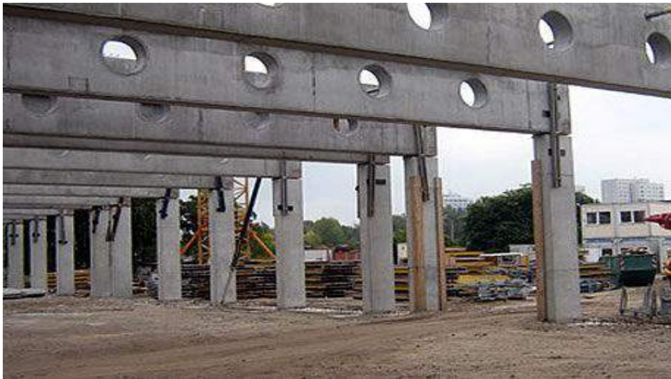
Plate (1.2) Prestressed concrete beams with opening [2] .
