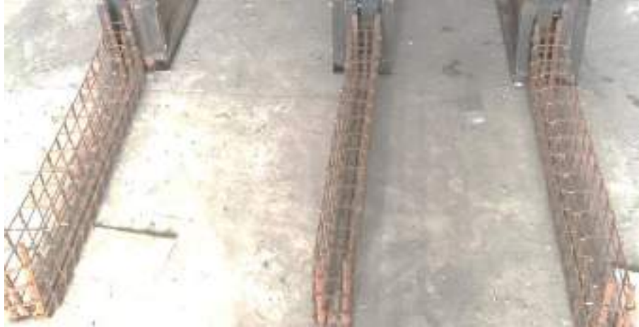
Plate (3.12) Steel reinforcement mesh.
