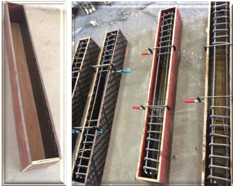
Fig. (3-14): Beam Molds and Reinforcement.
