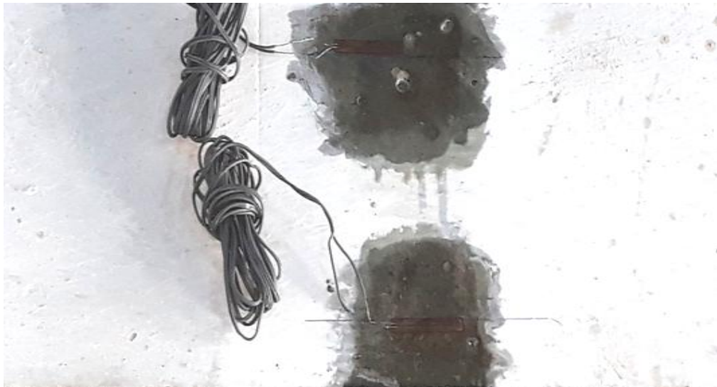
Fig. (3-20): Strain gauges attached to the beam
