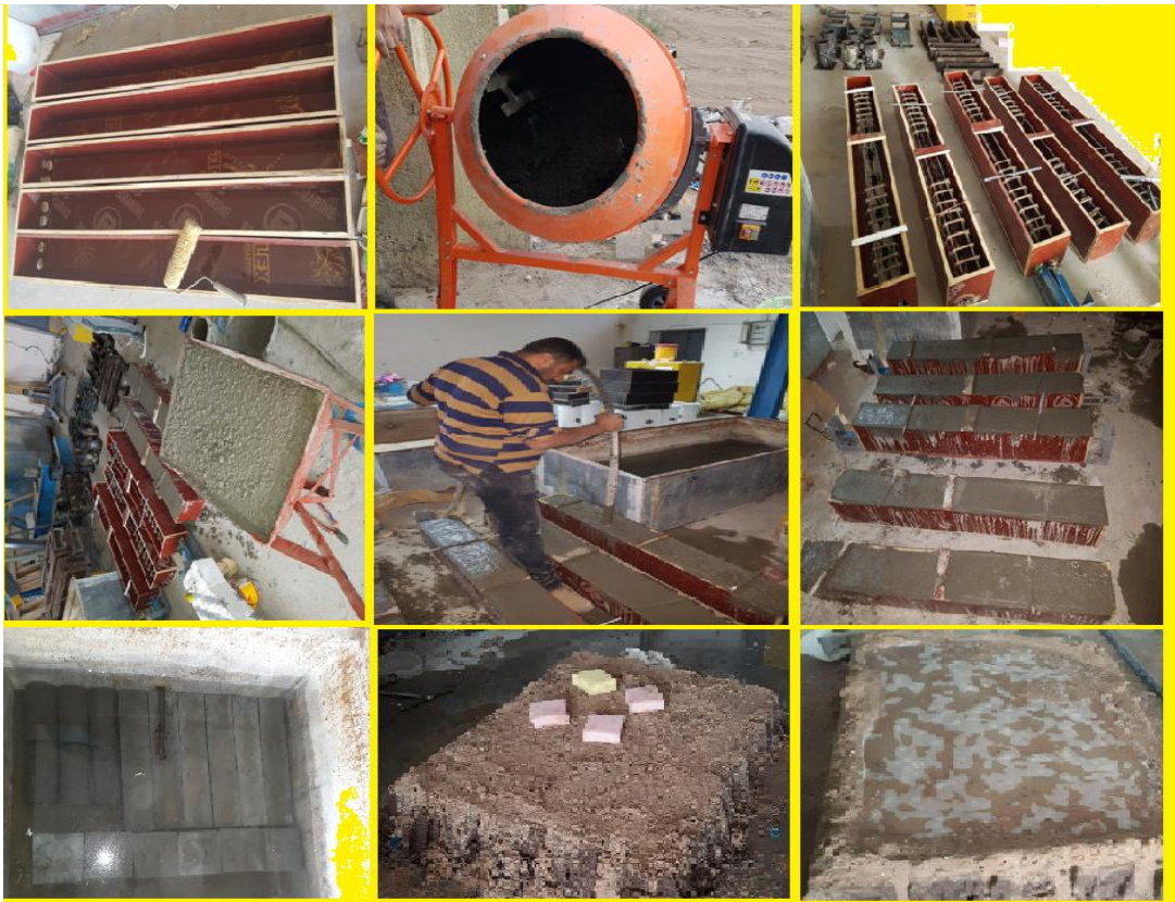
Fig. (3-37) : Preparing, casting, and curing for all beams
