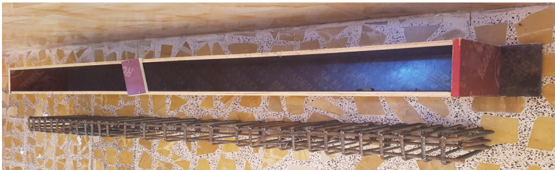
Fig. (3-16): Wooden molds for beams
