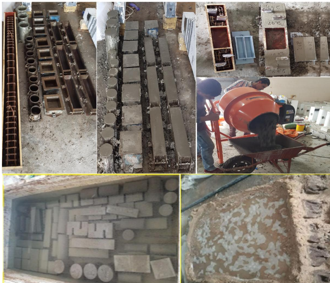
Fig (3-5): Preparing, casting and curing for beams and specimens
