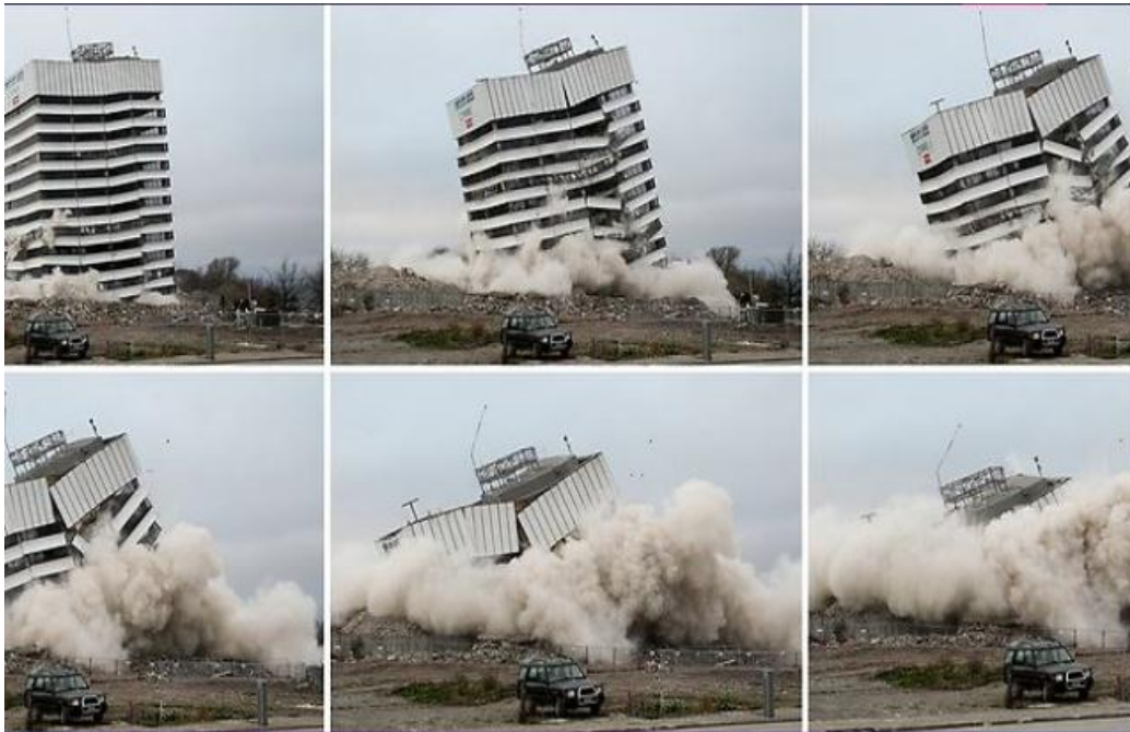
Figure (1-5): Building collapse due to wind load [8].
