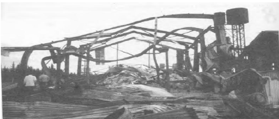
Figure (1-2): Steel structural failure due to fire [1].
