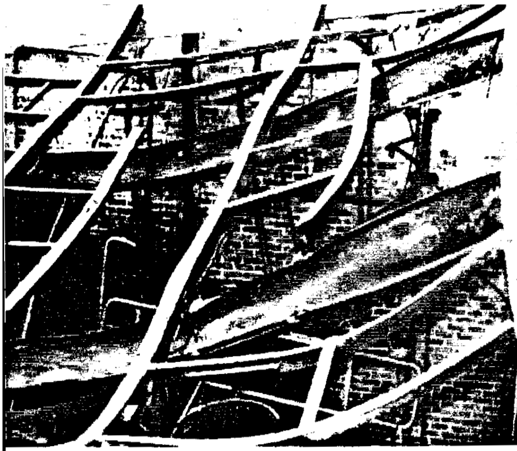
Figure (1-1): Deformation shape after fire [1].
