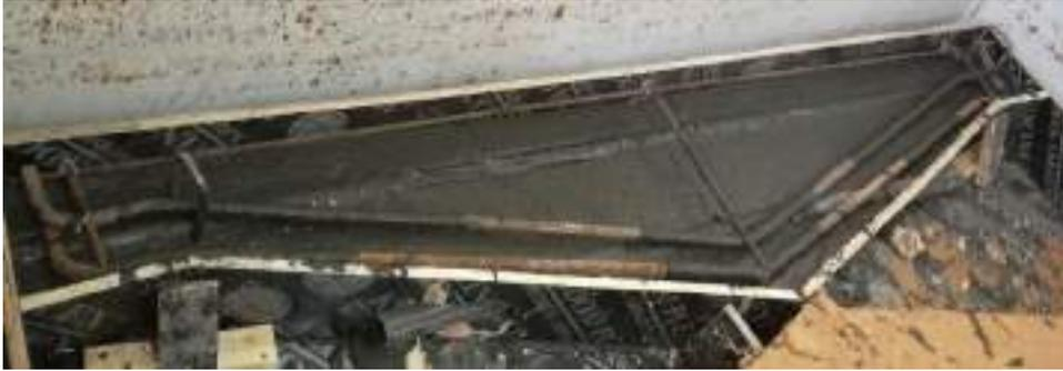
Fig 3-17 Casting of tapered-beam.
