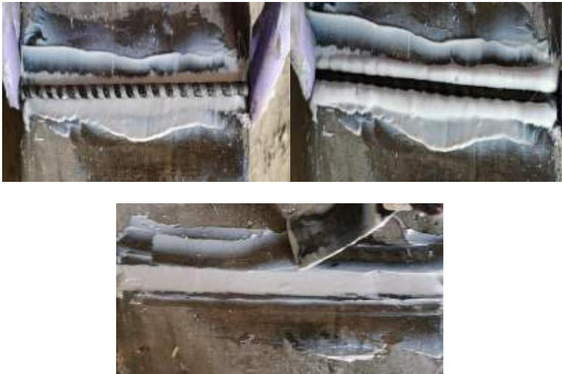
Fig. 3-25 Steps of NS CFRP bar installation.
