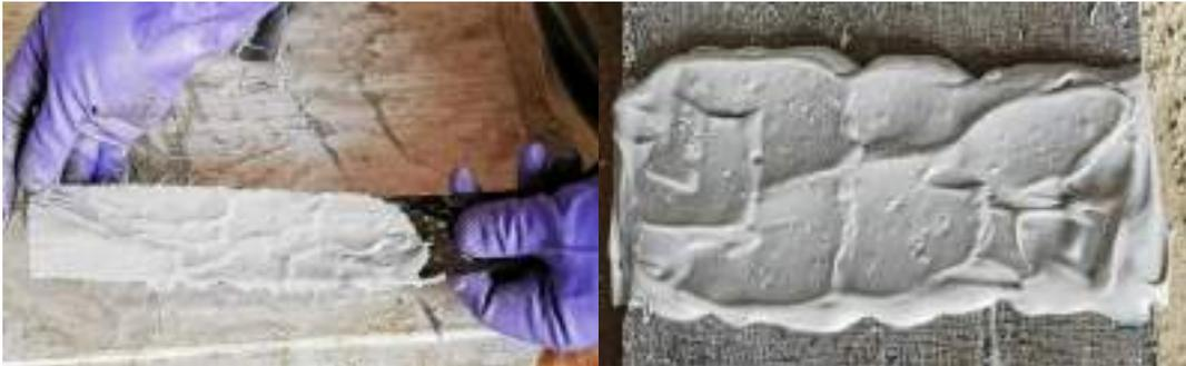
Fig. 3-26 Saturated of CFRP strips & concrete surface with epoxy.
