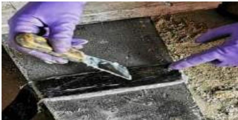
Fig. 3-27 Fixing of CFRP strip.
