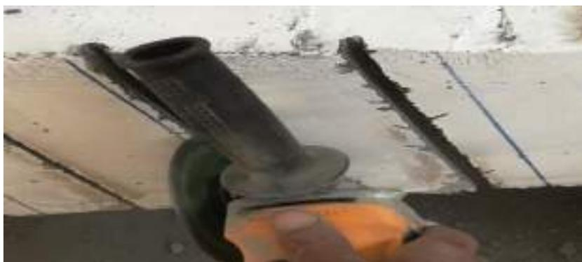
Fig. 3-24 Electrical diamond cutter to create grooves.
