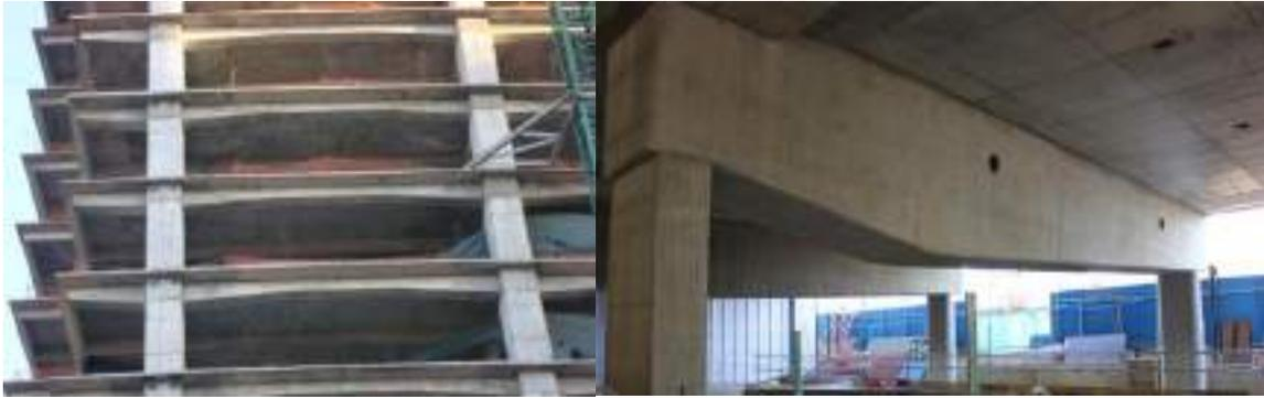
Fig. 1-1 Concrete tapered-beam [1].
