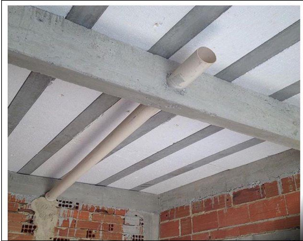
Figure 1.4: Service ducts and pipes in beams.
