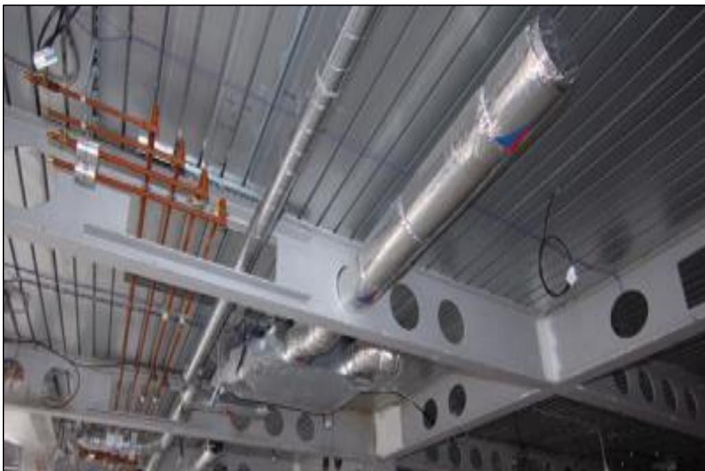
Figure 1.1: Service ducts and pipes in beams.
