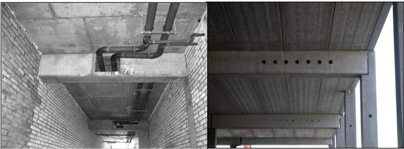
Figure 1.1 Examples explain the openings in beams [3].
