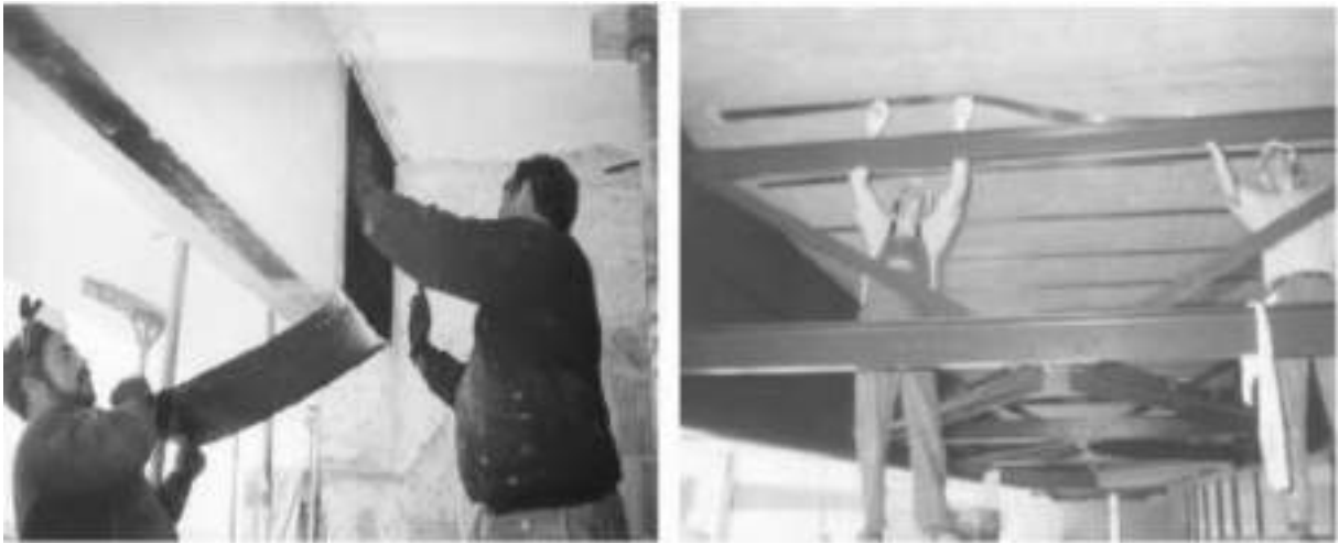
(a) Hand lay-up CFRP sheets.
