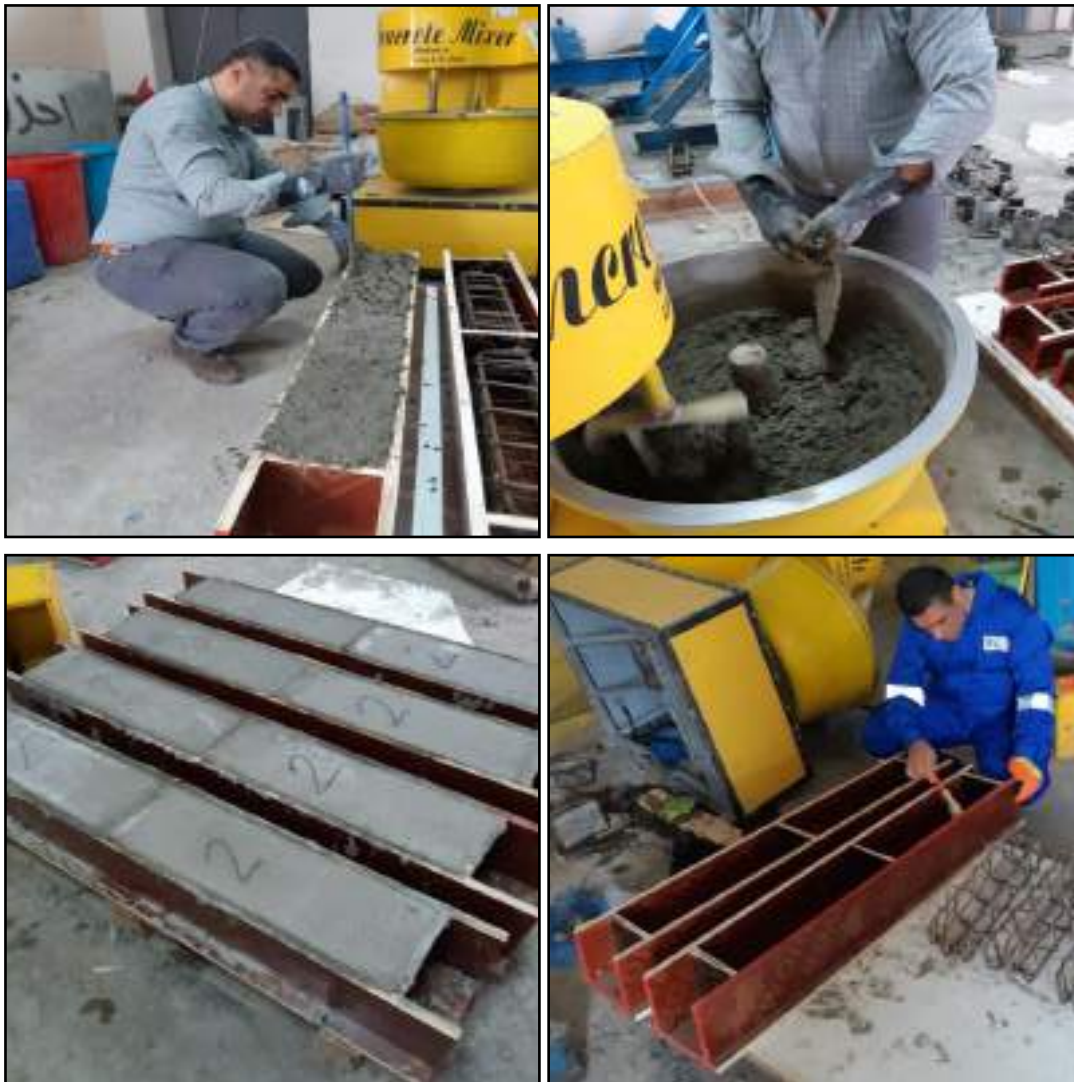
Figure (3-19): fabrication of the experimental columns.
