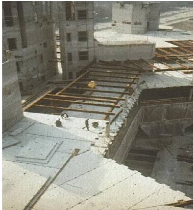
Figure 1.5 Use of Precast Concrete Floor Units [2].
