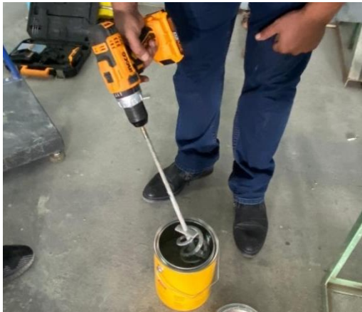
(c) Mixing of Sikadur - 52 LP epoxy
