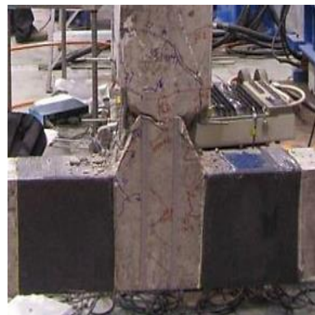
(b) Retrofitted specimen
