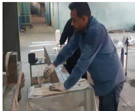
(f) Applying strengthening scheme
