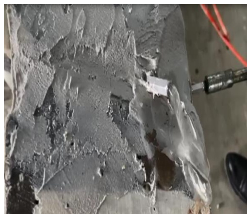
(e) Inject of the viscosity resin epoxy Sikadur - 52 LP
