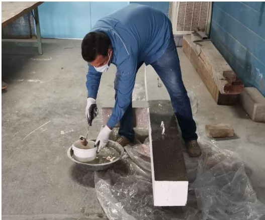
(c) applying layer of primer epoxy
