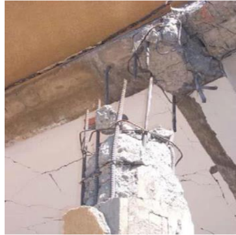
(a) Un adequate anchor
