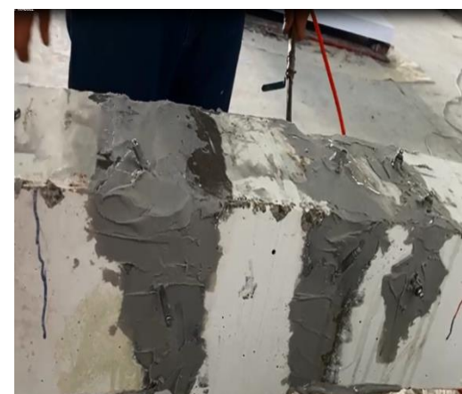
(f) Close the needles and packers
