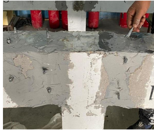
(b) Close the cracks and damaged area around the injection needles
