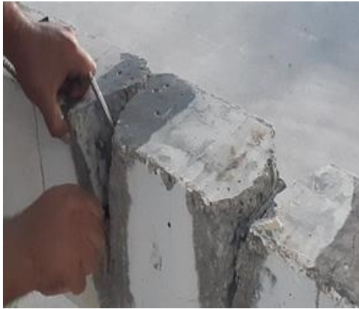
(a) Install the injection needles and packers
