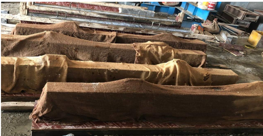
Figure 3.17 The Details of Beams Casting.
