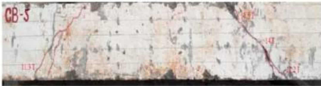
Fig.(2-3): Crack pattern for control beam [40].
