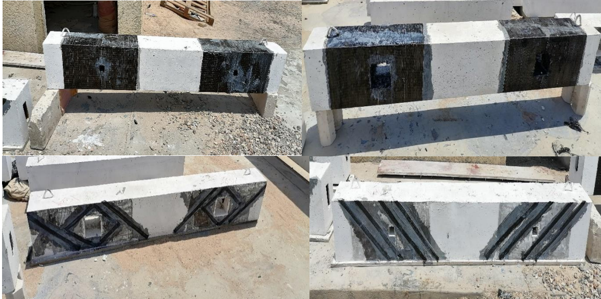
Figure 3.29 Composite encased steel-concrete beams with square openings strengthened by CFRP strips.
