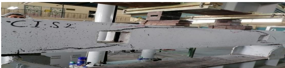
Figure 4.5 Load-deflection behavior and crack patterns for CIS2.
