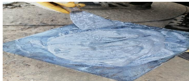
Figure 3.27 Light gray paste of Sikadur®-330 components (A+B) mixing.
