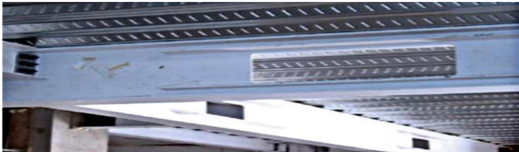
Figure 2.9 Rectangular web openings in composite beams[64].
