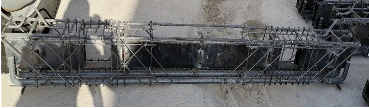
Figure 3.15 Large transverse square openings strengthening by reinforcement arrangement RIS2.
