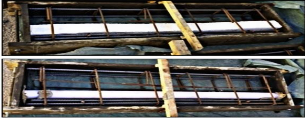
Figure 2.15 Casting beams with the longitudinal opening[72].
