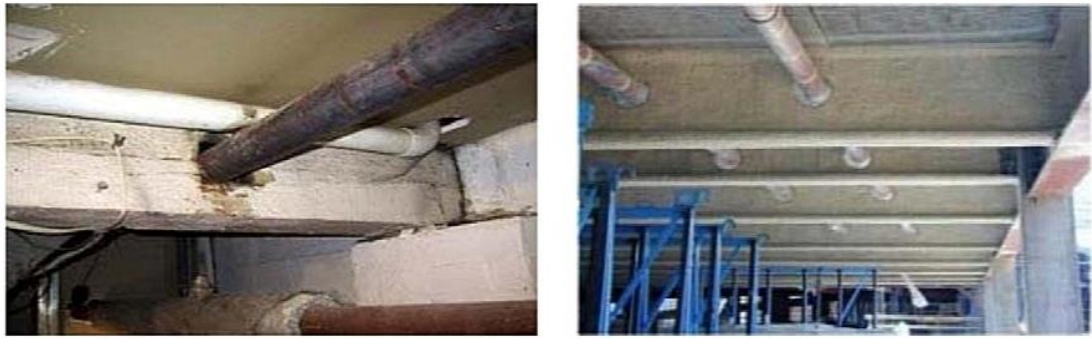
Figure 2.16 Beams with openings[73].
