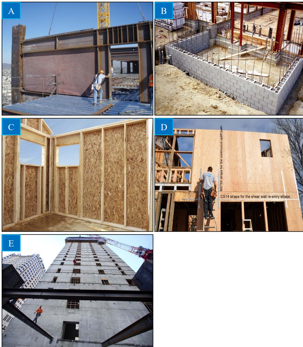
Figure 1.4 Shear walls classification by material (A) steel plate, (B) reinforced concrete hollow block masonry, (C) mid-ply, (D) wooden, (E) reinforced concrete.
