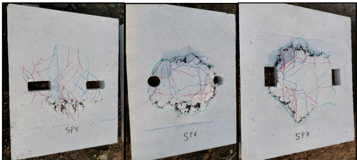
(c) Crack patterns for tested slabs group A2
