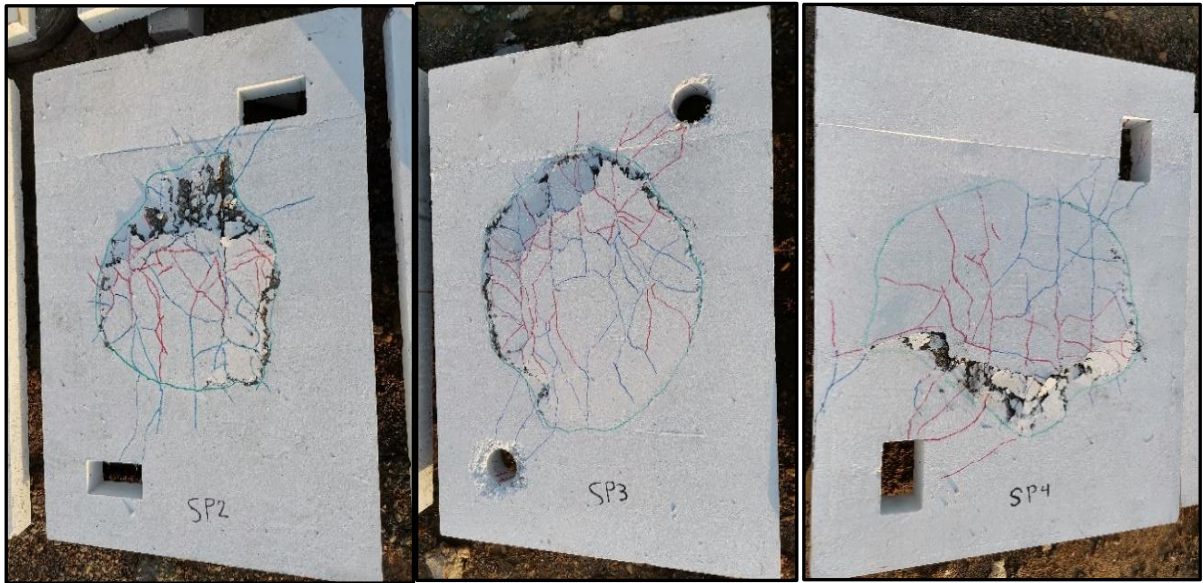
(a) Crack patterns for tested slabs group A1
