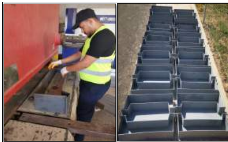
Figure 3.18 The Constructed Formwork.
