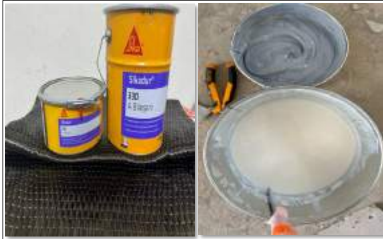
Figure 3.12 Mixing Two Components of Epoxy Resin.
