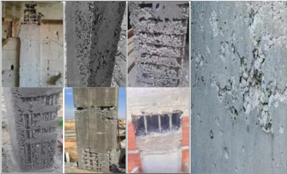
Figure 1.7 Honeycomb in Columns.
