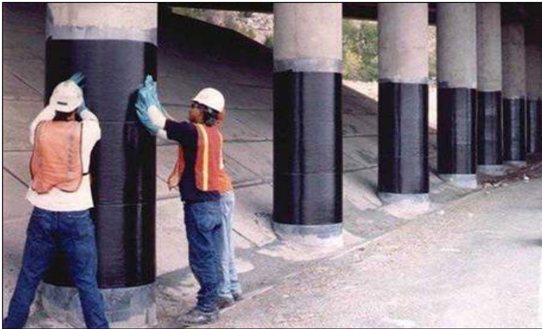
Figure 1.5 Details of CFRP Jackets Technique.[12]
