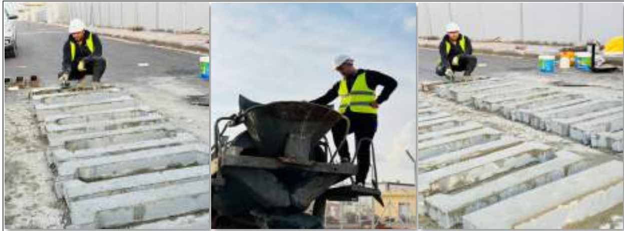
Figure 3.21 Pouring and Compacting Process of Concrete.
