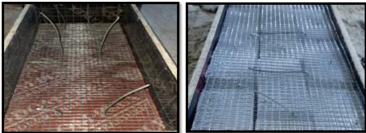
(c) Shear connectors at top.
