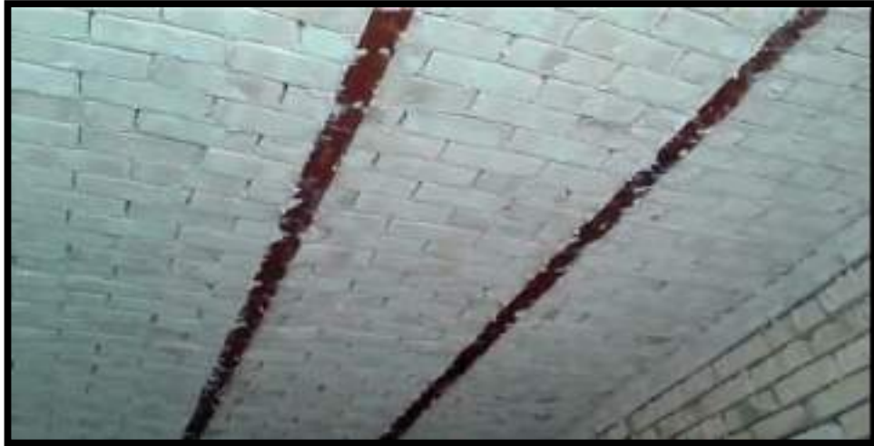
Figure. 1-1: Jack arch slab after construction.
