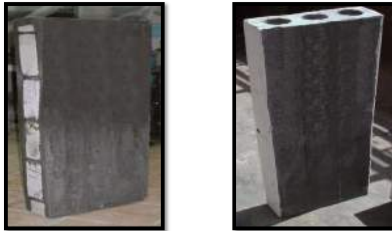
(a) Lightweight brick sandwich panel. (b) Hollow core panel.
