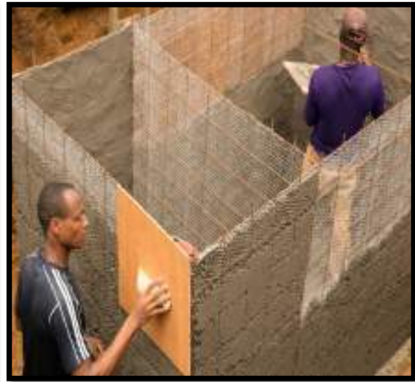
(b) Construction septic tank [13].
