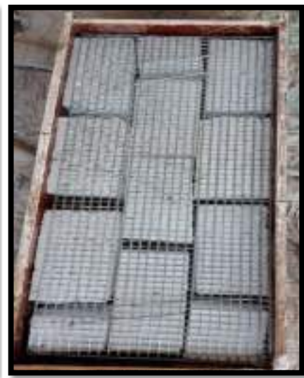
(c) Apply reinforcement cage for top layer.
