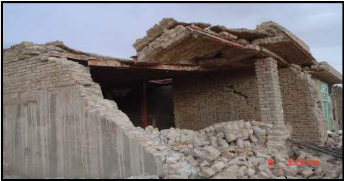
Figure. 2-2: Failure modes of masonry structures [8].
