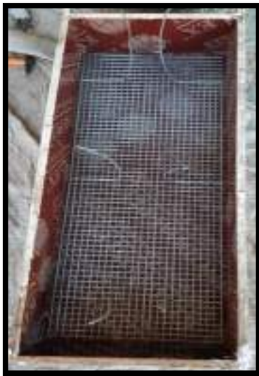
(a) Prepare mold and reinforcement cage for bottom layer.
