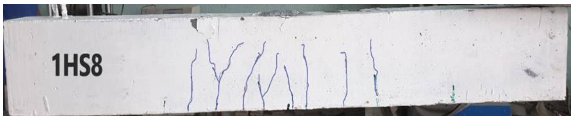
Figure 4.29 Flexural failure for beam 1HS8.
