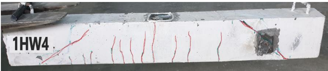
Figure 4.36 Flexural-Shear failure for 1HW4.
