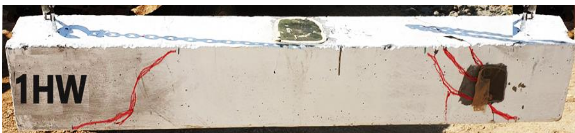
Figure 4.34 Diagonal shear failure for beam 1HW.
