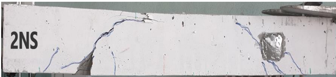
Figure 4.25 Diagonal shear failure for beam 2NS.
