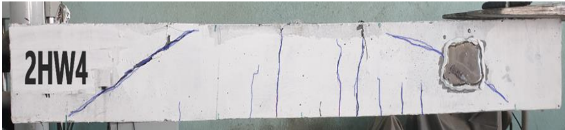
Figure 4.35 Flexural-Shear failure for 2HW4.
