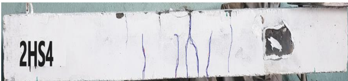
Figure 4.26 Flexural failure for beam 2HS4.
