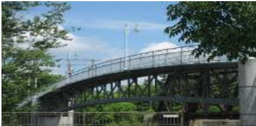
Fig. (1.4) Sherbrook Pedestrian Bridge, in Canada.
