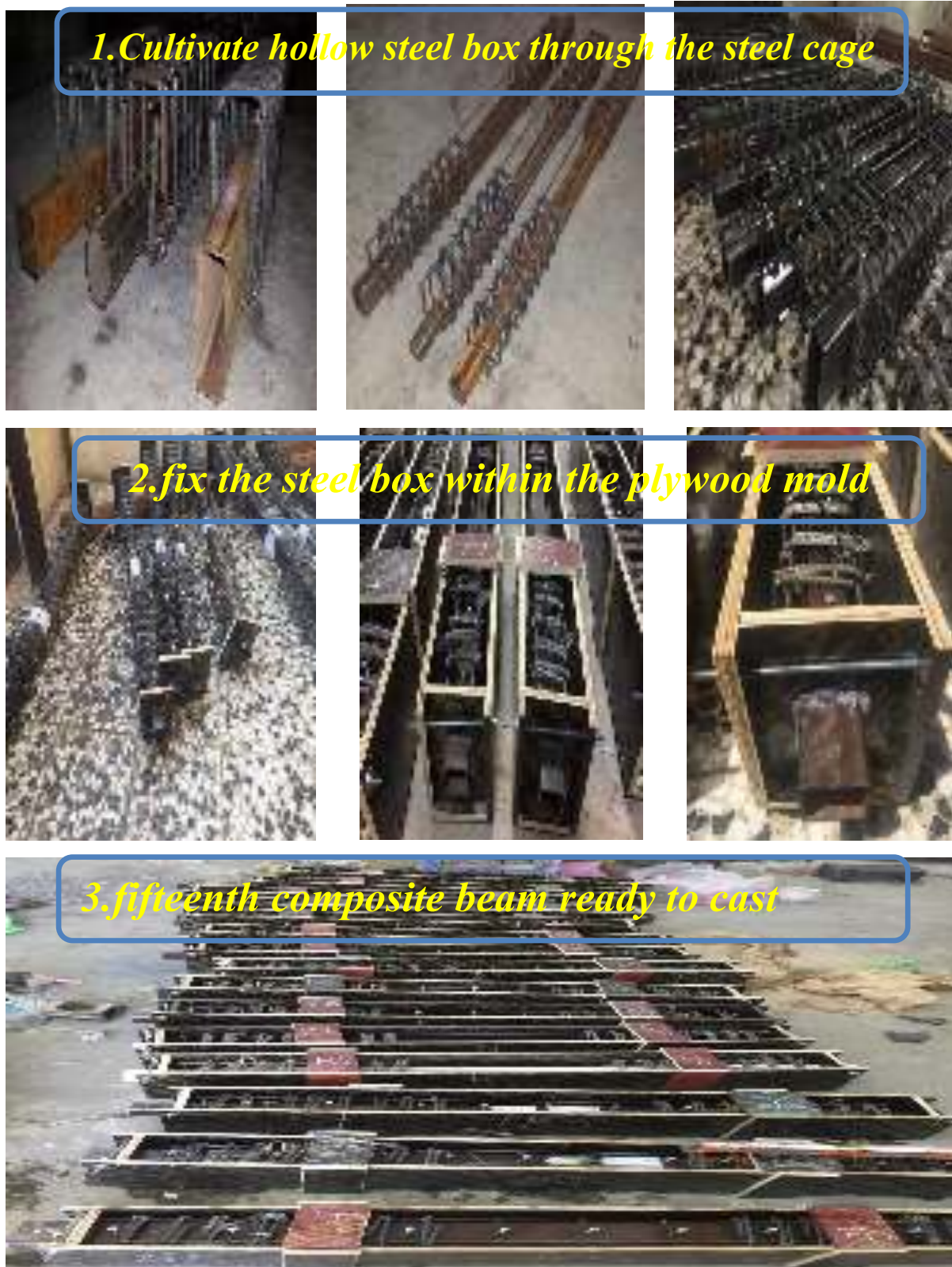
Plate (3.9) Installation steel box and fixed it.
