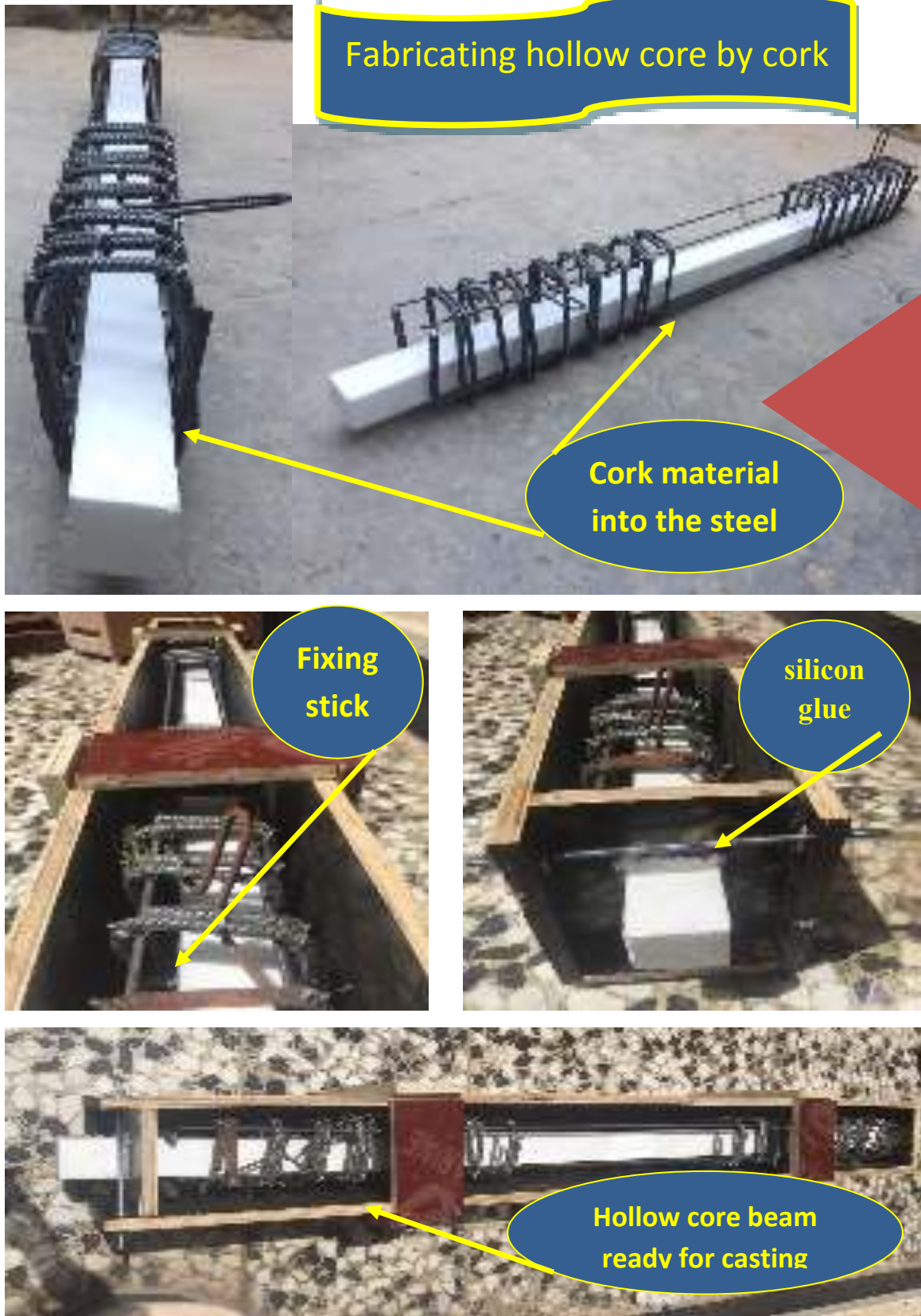
Plate (3.8) Preparing the opening mold for the hollow beam(B2).
