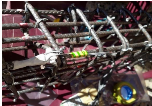
c. adhesive strain gauge of steel on reinforcement
