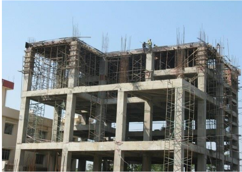
Figure 1.2 Structural members of reinforced continuous concrete buildings [7]
