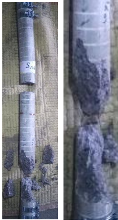
Plate (4.5) Failure mode of slender concrete column SA4
