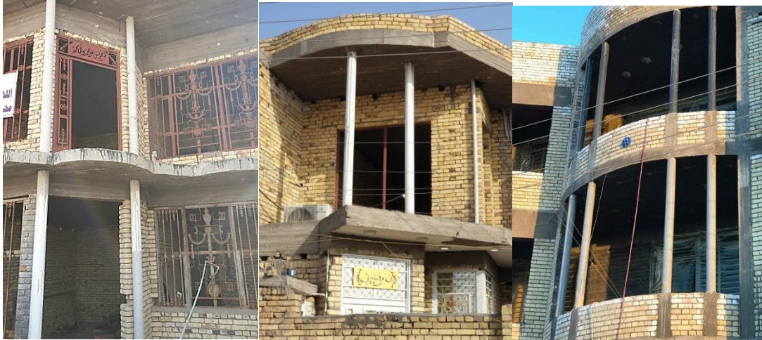
Plate (1.1) Using the plastic tubes as a formwork and for aesthetic.
