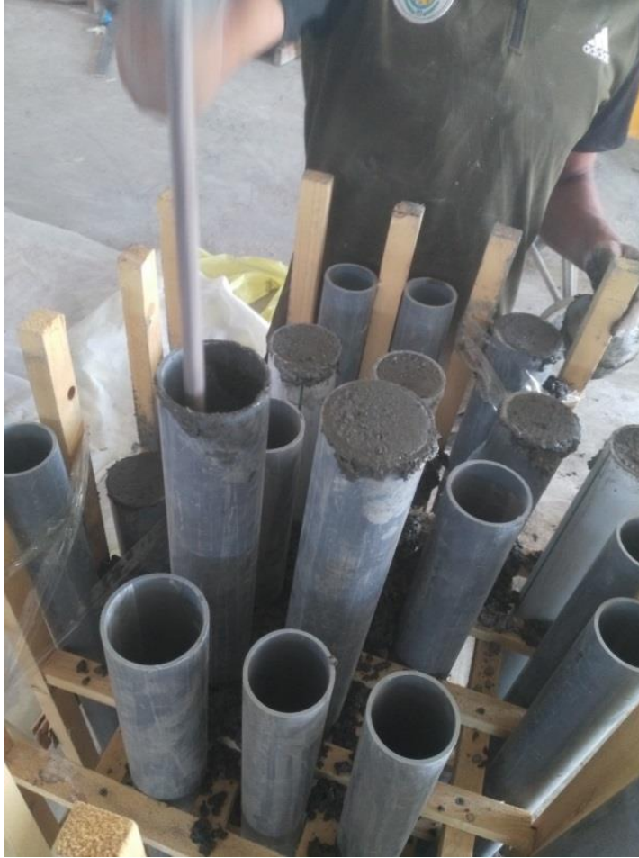
Plate (3.9) Casting column specimens.
