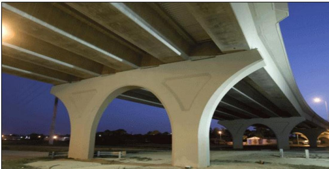
Figure 1.4 The North Boulevard Bridge in Louisiana was made from high strength concrete (de Rooij & Mendonça Filho, 2015).
