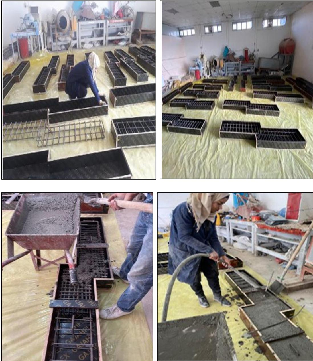
Figure 3.20 Pouring and processing beams.
