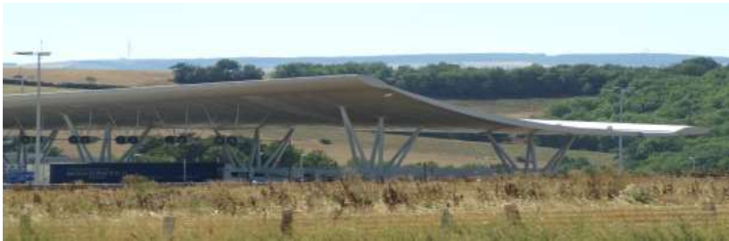
Figure 2.2 Toll-Gate Millau Viaduct in France[11].
