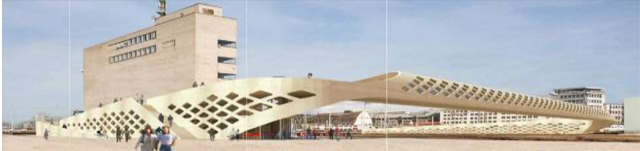
Figure 2.10 Negrelli-Pedestrian Bridge, Main Railway Station-London[11].
