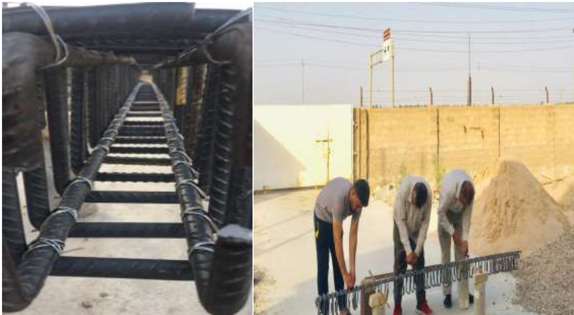
Figure 3.7 Beam Reinforcement.
