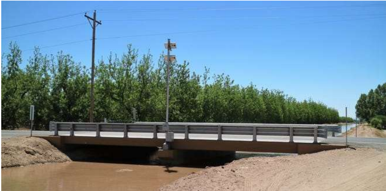
Figure 1.1: Two span bridge from UHPC in Anthony, New Mexico [4]
