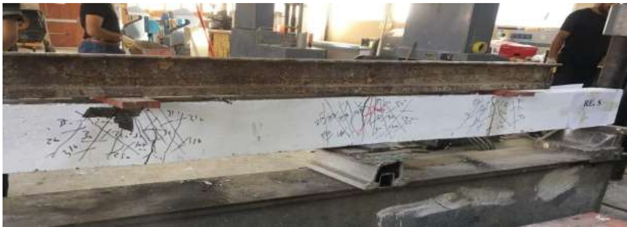
Figure 4.11 Crack pattern of solid beam-RE.S (1.5% S.F).
