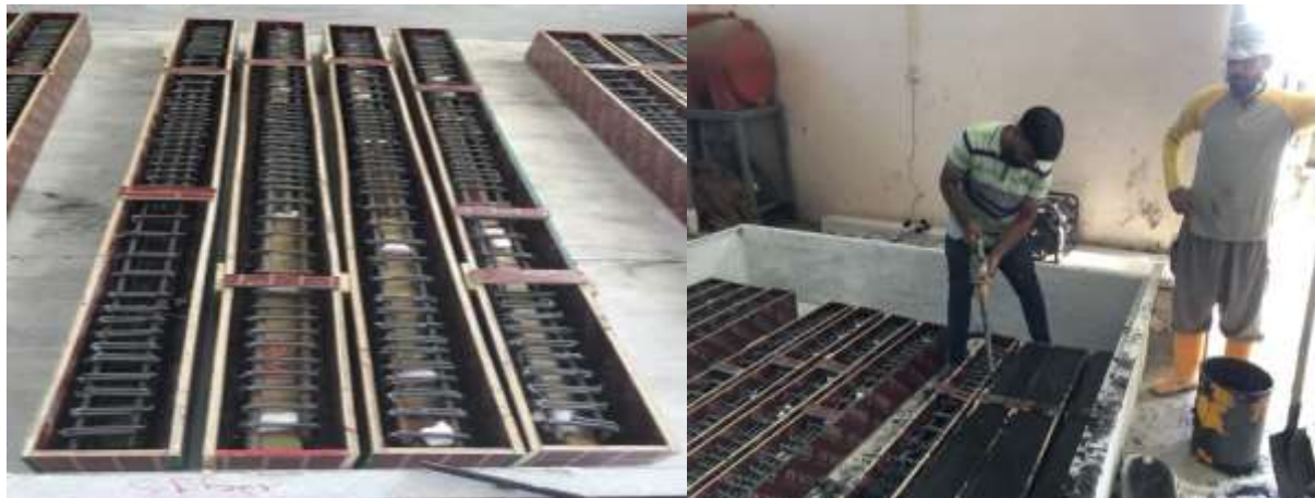
Figure 3.12 The steel bars in required position.
