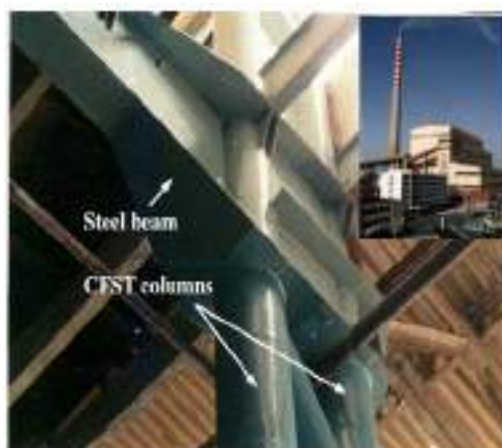
Figure (1- 3) A power plant workshop using CFST columns
