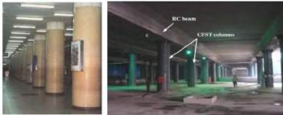
Figure (1- 2) Subway stations (Beijing Metro) using CFST columns
