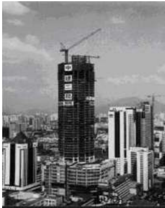
Figure (1- 4) SEG Plaza highest building adopted CFST (under construction)
