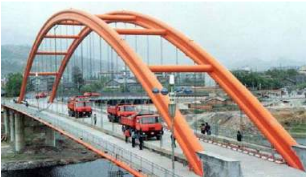
Figure (1- 5): First CFST Arch Bridge, China: Wangchang East River Bridge (Span 115 m)
