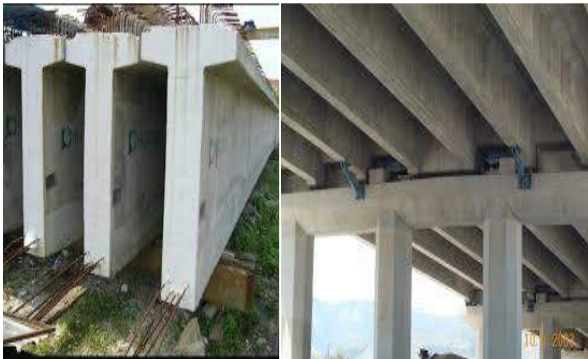
Figure (1-2) T-Beam member[2]
