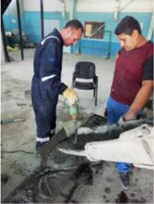
Figure ( 3-15 ) Compaction process
