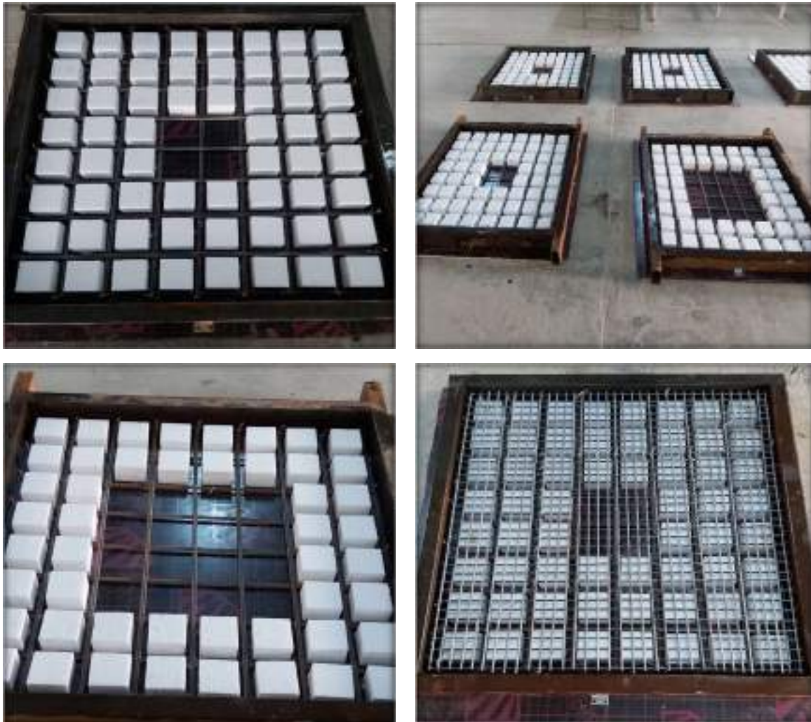
Figure 3. 16 Specimens molds, waffle blocks, and steel reinforcement.
