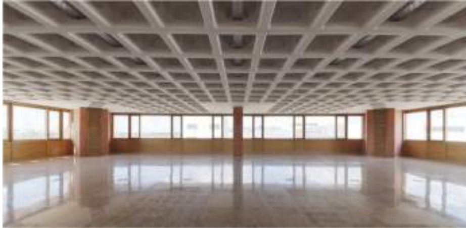
Figure 1. 4 Waffle Slab Structural Floor System.
