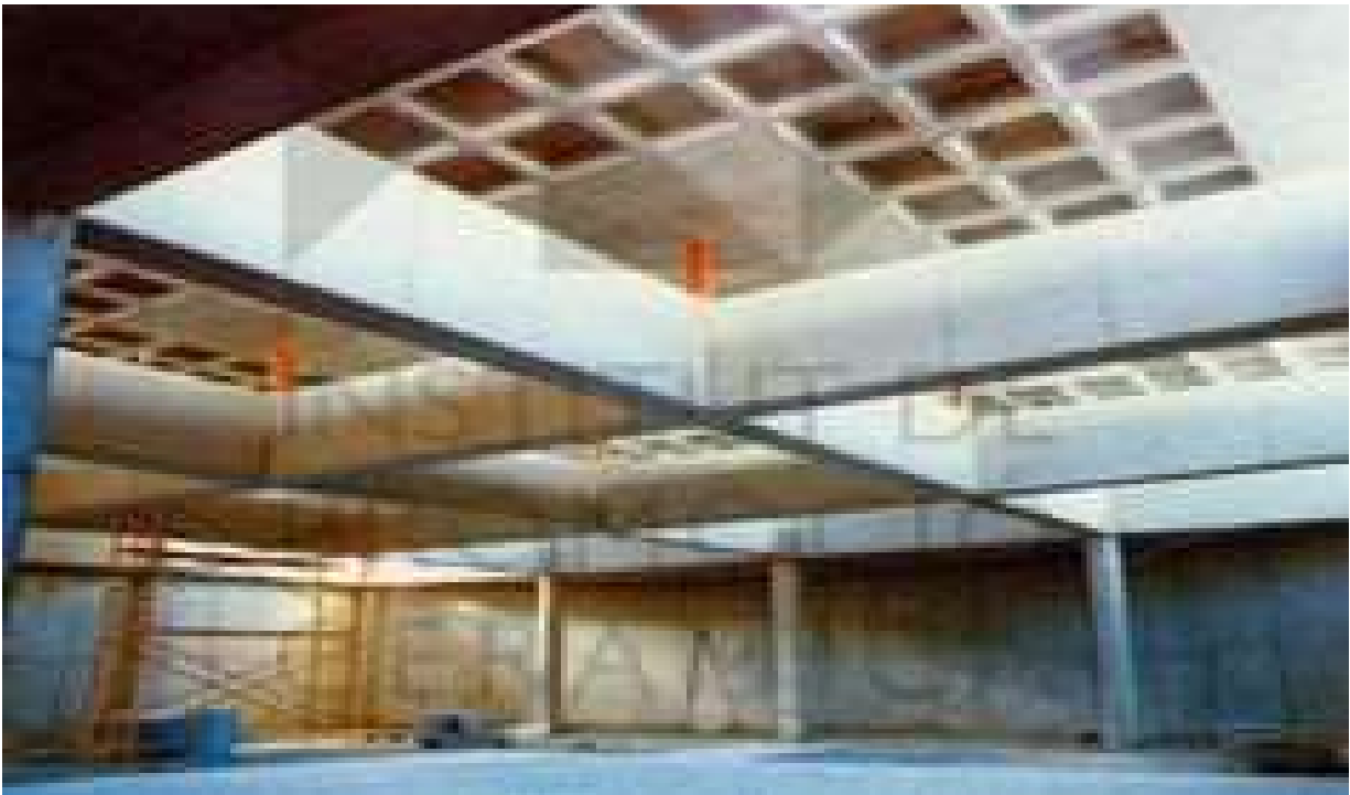
Figure 1. 6 A Waffle slab with dimensions 20 * 20 - a fire station at San Vicente city in Spain [16]
