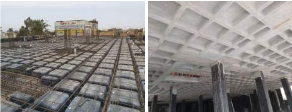
Figure 1. 5 Hybrid configuration of waffle slab.
