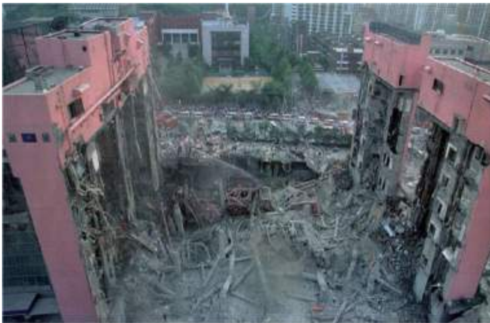
Figure 2. 1 Collapse of Sampoong commercial store [28].
