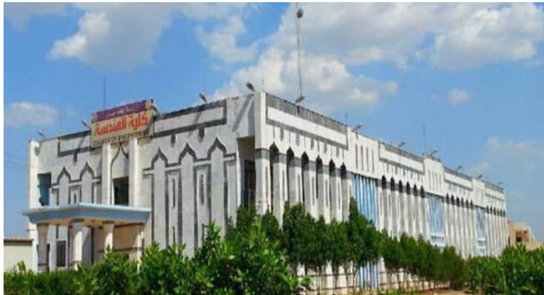
Figure 1. Building case study
