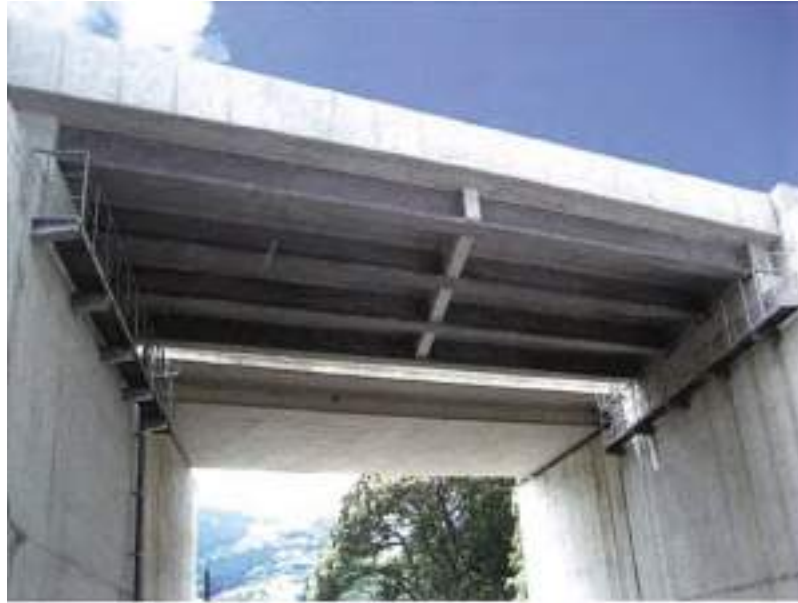
Figure 1-2: The Horikoshi C ramp bridge in Japan (Resplendino and Toulemonde, 2013).
