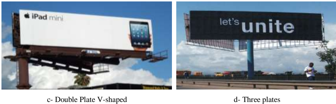
Figure 1. Large billboards configurations.
