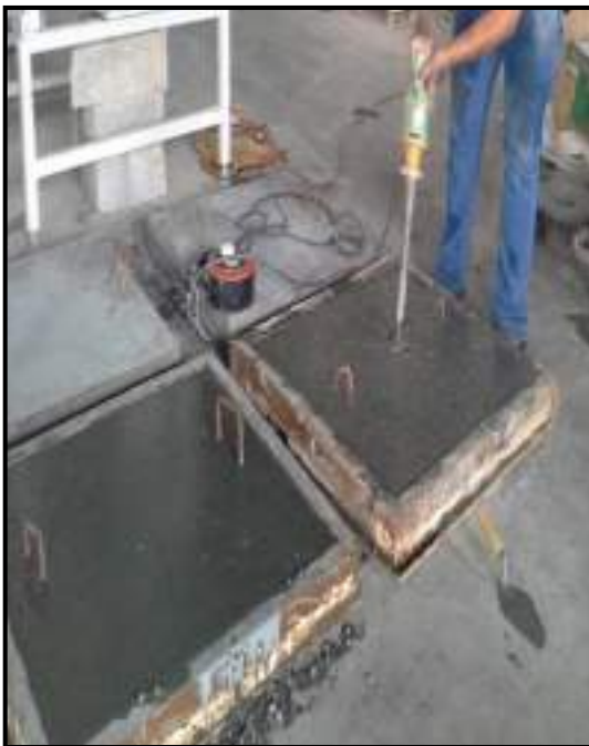
c - Compacting process
