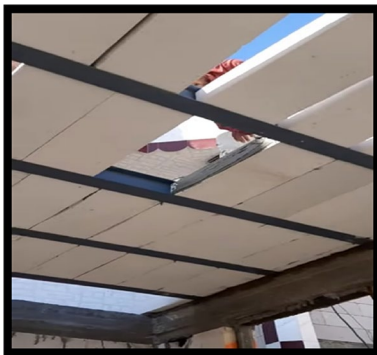
Fig. 1 Construction of a jack arch slab by cellular concrete blocks
