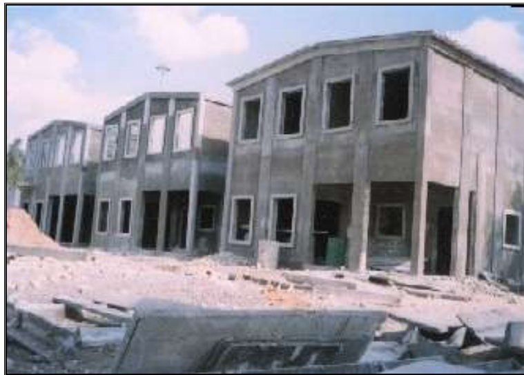
Plate (1-2) Two story house units under construction in Baghdad [10]
