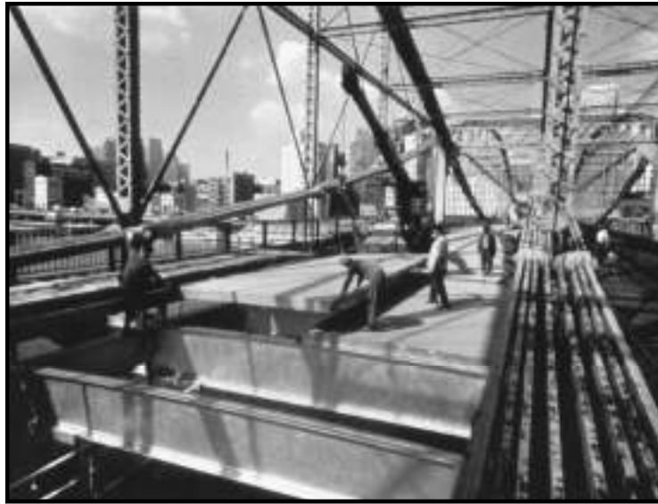
Plate (1-1) Installation of an aluminum deck on aluminum beams [5]
