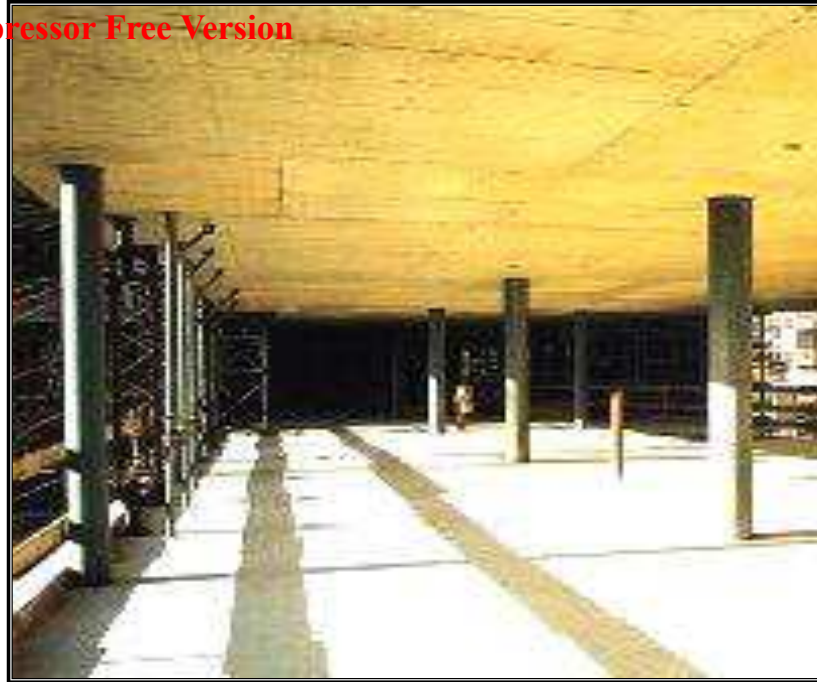
plate(1-1): Flat Plate Construction[3].
