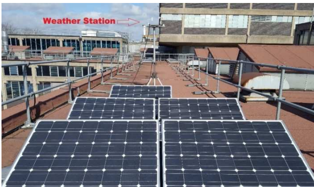
FIG. 1. THE ROOF-TOP PV SYSTEM BUILT-UP AT THE LABORATORIES OF BRUNEL UNIVERSITY LONDON, UK.
