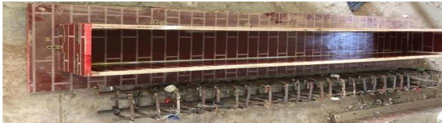
**FIGURE 5.** Wooden molds for beams.
