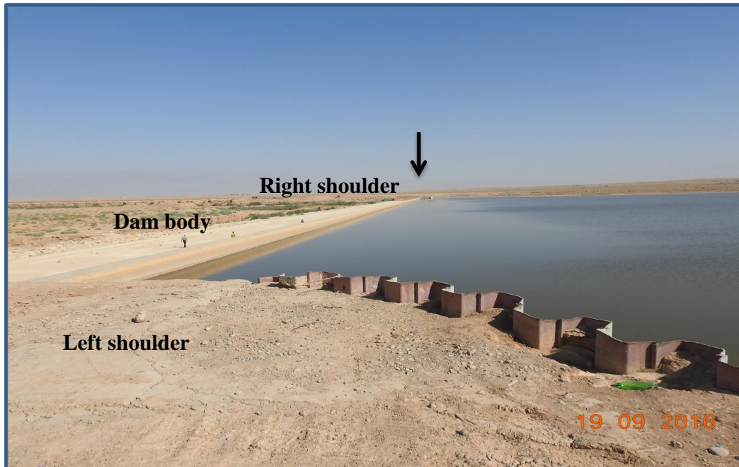
Fig.3.15 Dam site (in August,2016)
