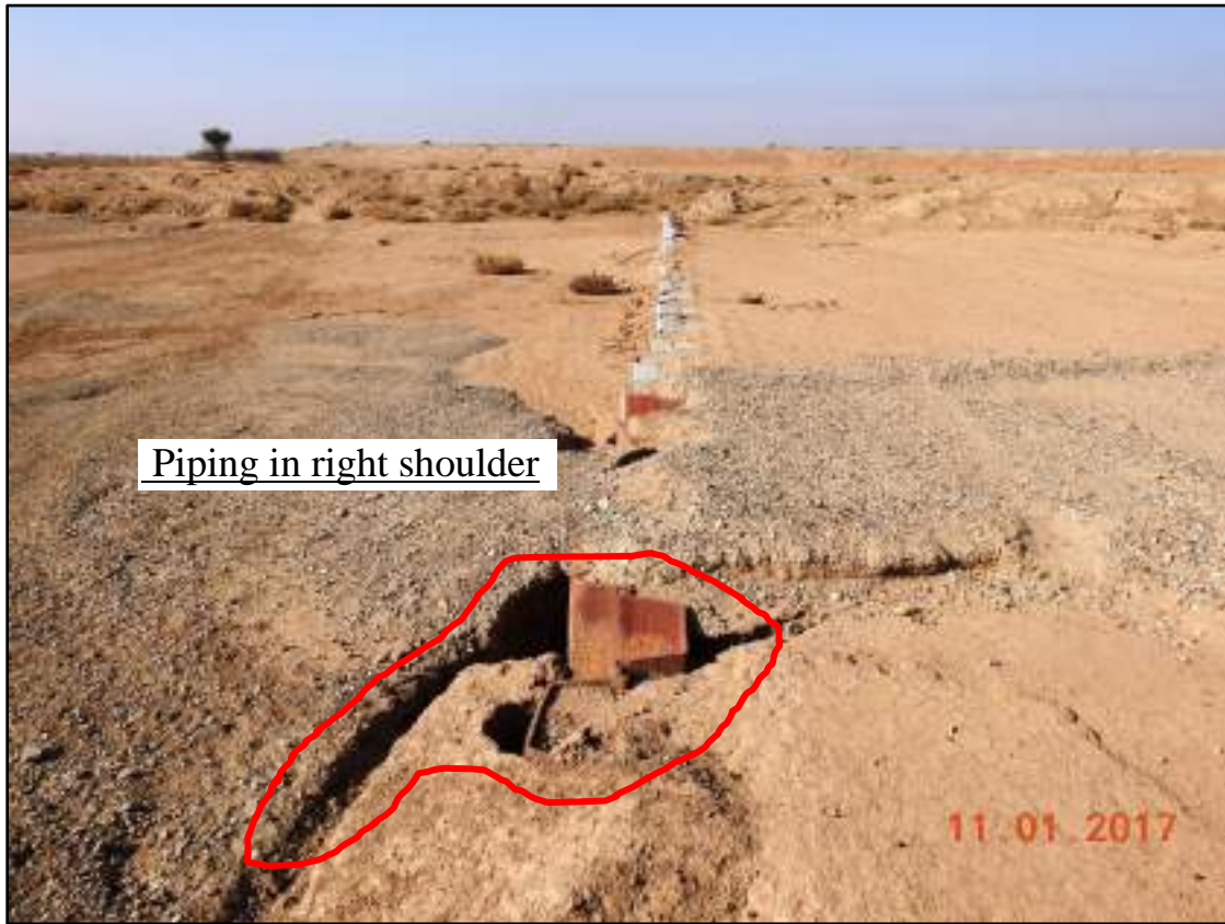
Fig. 5.18 Cavity & hole by the action of dispersion
